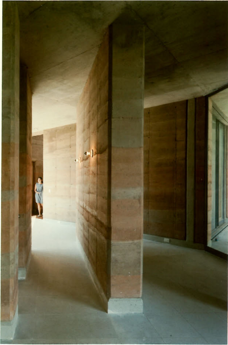
Right, a model shows the precise configuration of the house with its angled roofs and two main sections. Above, an interior view showing the use of rammed-earth walls.
